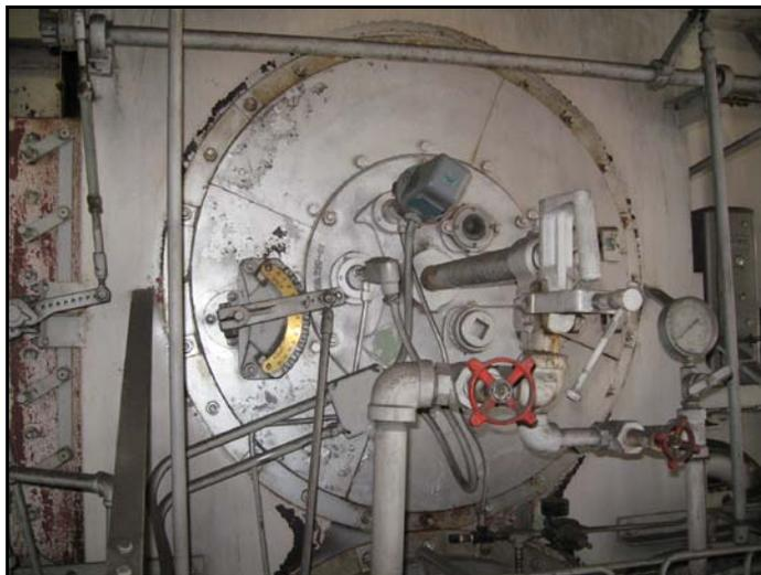
Boiler Nos. 2 through 4 can generate 60,000 pounds per hour (PPH) of steam when firing natural gas or No. 2 fuel oil; and Boiler No. 1 can generate 30,000 PPH of steam utilizing natural gas or
